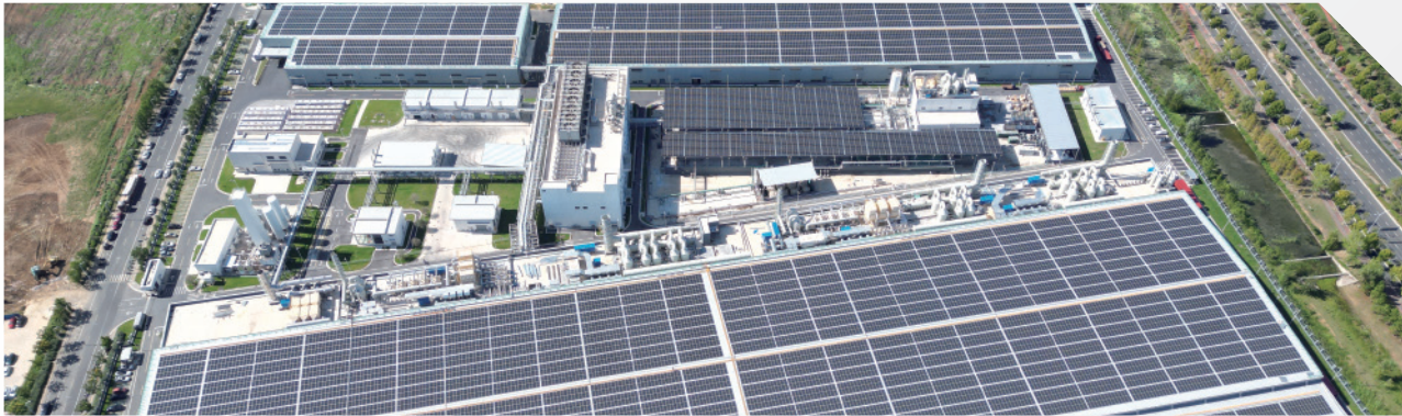
10.2MW 📍 Project Location: Chuzhou, China 📋 Module Type: Solar N Plus N-Type 575W 🕒 On-grid Date: 2024.10
